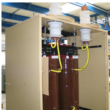
Single-phase transformer for excitation of 1,350 kVA, 22 kV generator;
