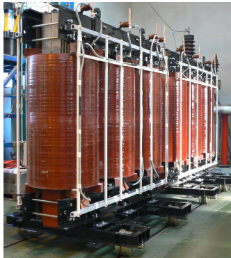
8000kVA transformers with 20/6kV ratio;
