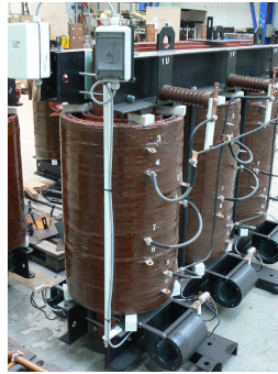
630kVA transformer with 15/0.4kV ratio and AF cooling system;
